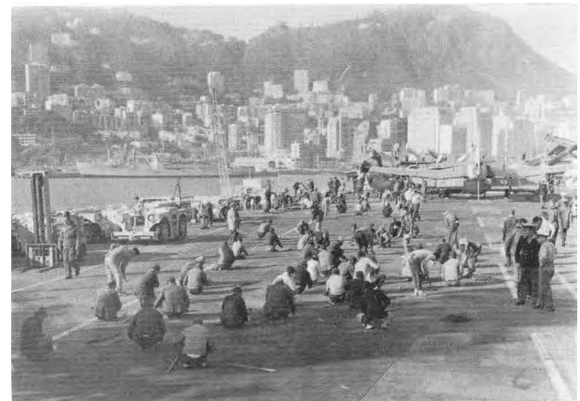
Chinese contract labour chipping the Flight Deck
